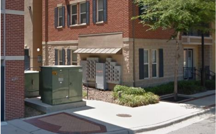
Prohibited (not facing the street, but still visible)
