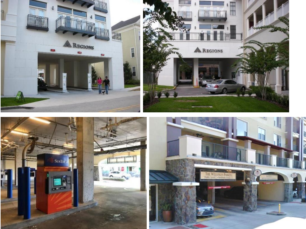
Figure XIV - 44. Interior Drive-Through Facilities
