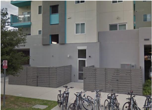
Allowed (utilities screened by fence)
